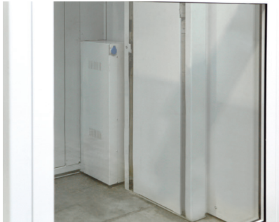
MRL Solution, control and pump unit inside the shaft.
